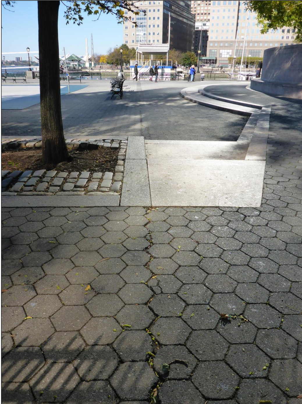
Photo 5 - View of paved esplanade above the joint between the platform and bulkhead. Note: Minor separation of pavers, no visible subsidence. Photo taken from Bent 81 looking north.
