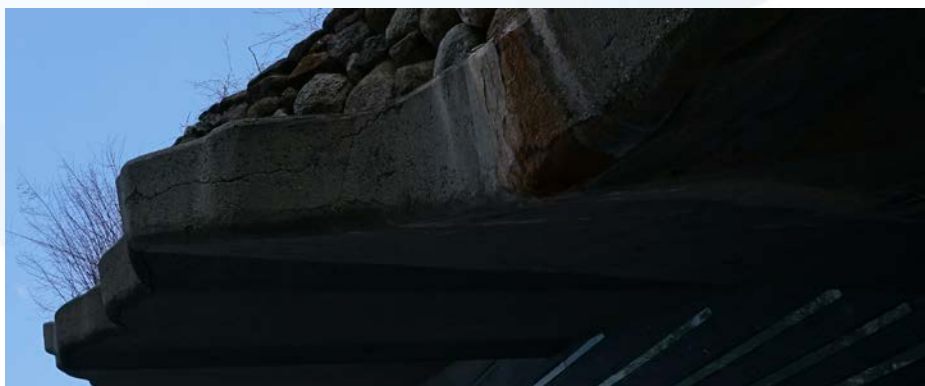
Figure 2: Horizontal cracking was present on the lateral surface of the cantilevered soffit.
