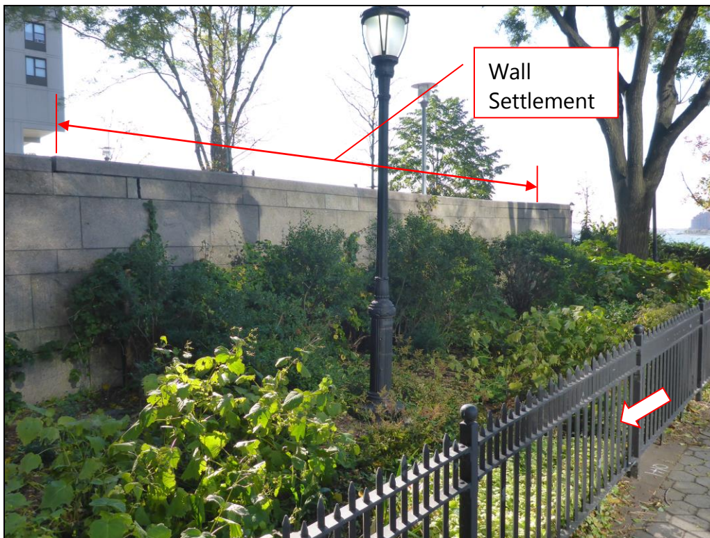
Photo 2 - Esplanade above Bents 80-81. Note settlement of wall and sinkhole (see arrow).
