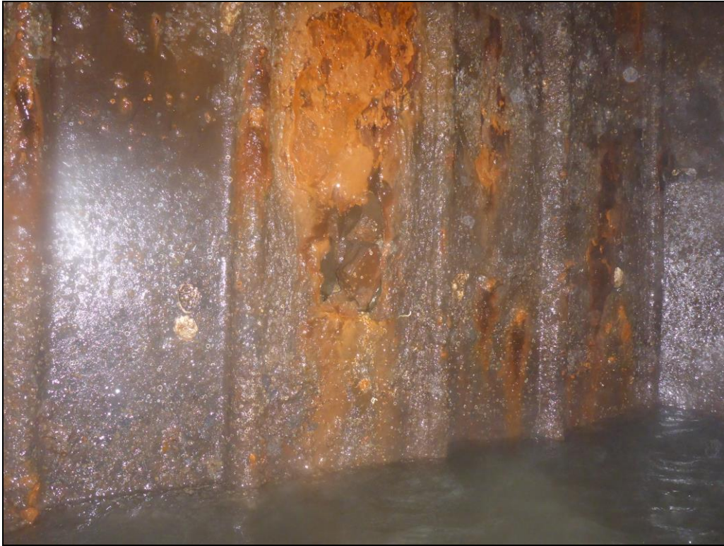
Photo 3 – Holes #1 & 2 in sheeting at Bent 81. Note additional corrosion of steel above hole.
