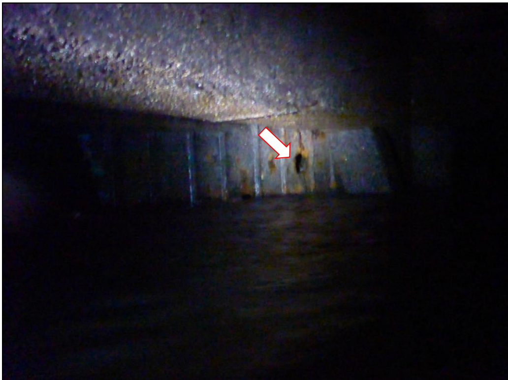
Photo 4 - Hole #4 in sheeting at Bent 87, void with fill loss visible during inspection.
