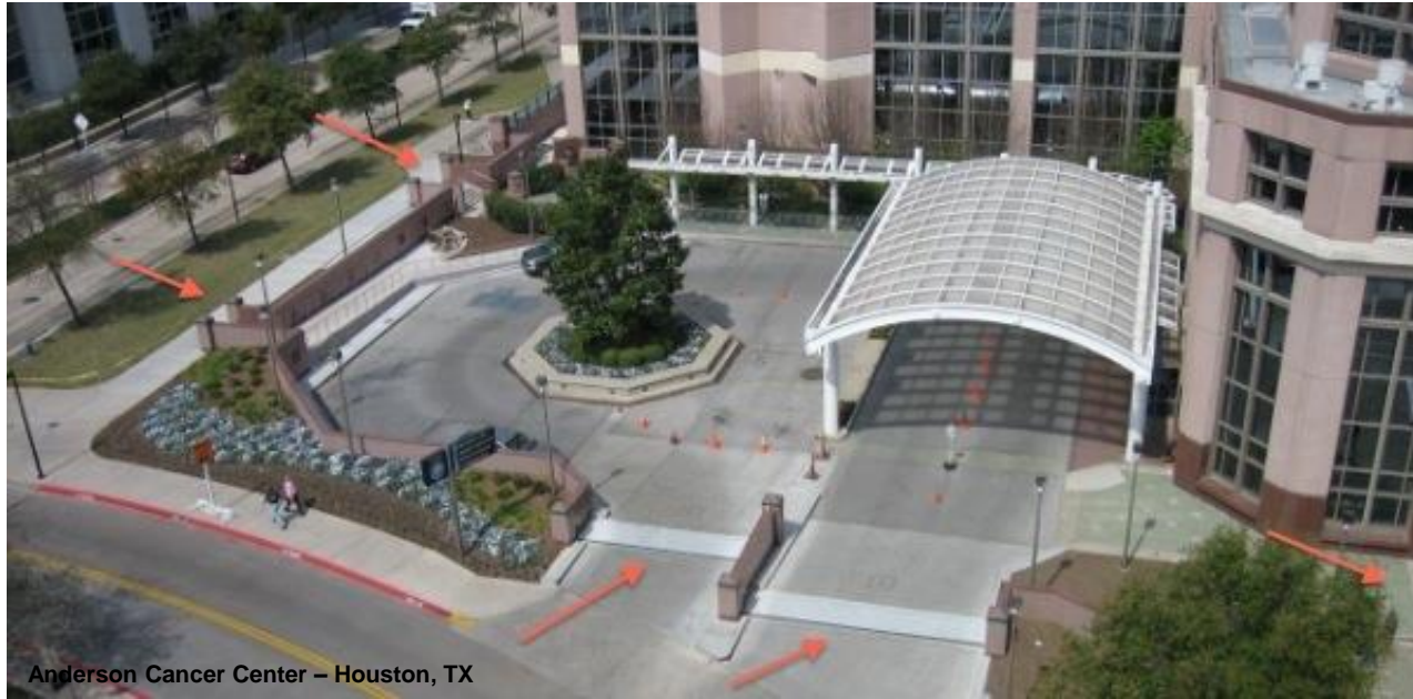
Passive flood barriers combined with garden walls
