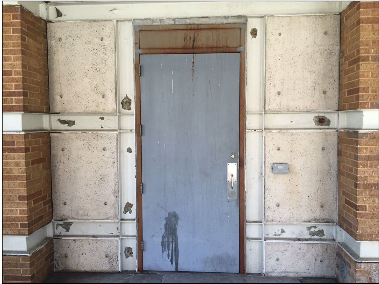
EMBEDDED STEEL CHANNELS IN EAST AND WEST STAIRWELL LANDING AND ADJACENT BUILDINGS
