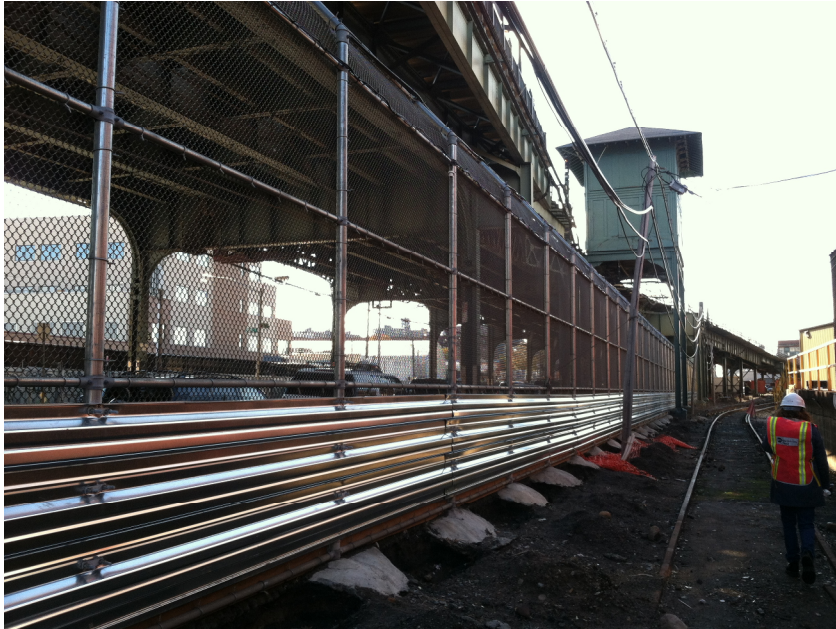
Metal deck fence protection at Coney Island Rail Yard
