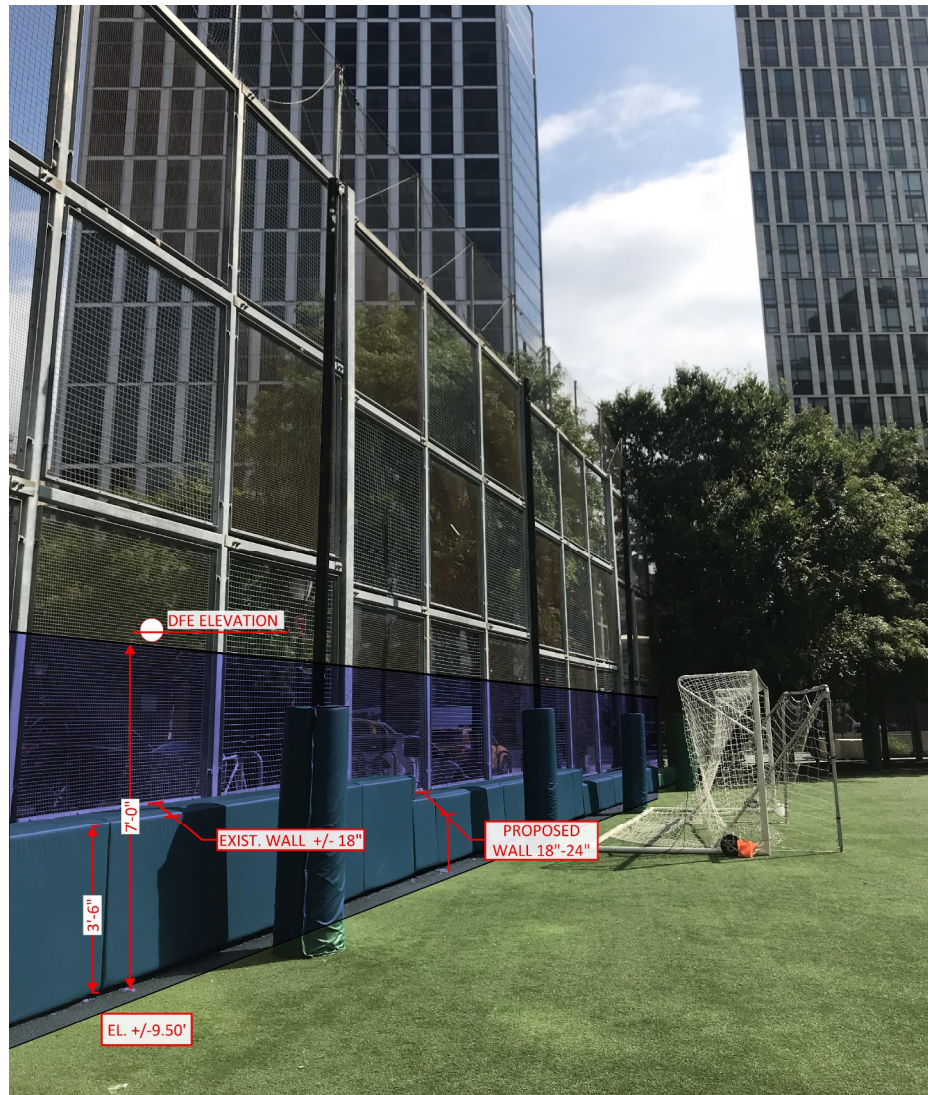
Looking Northeast along Warren St.
