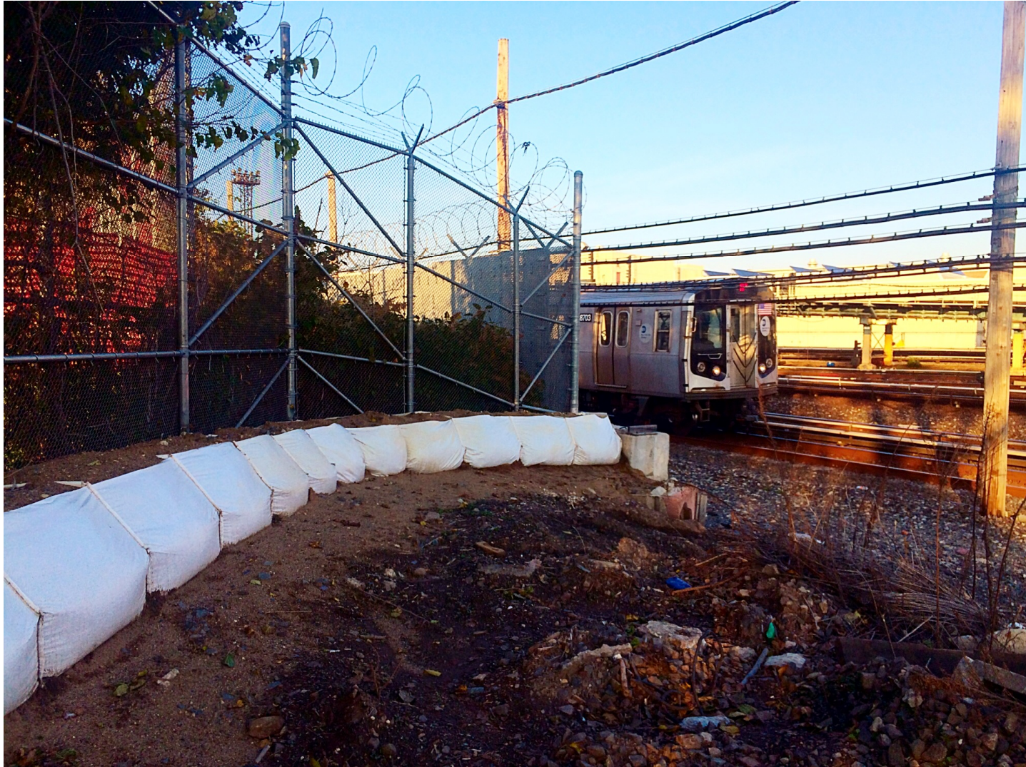
Trapbag protection at Coney Island Rail Yard
