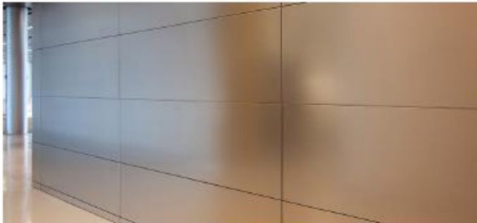
UNPAINTED STEEL WALL PANEL
