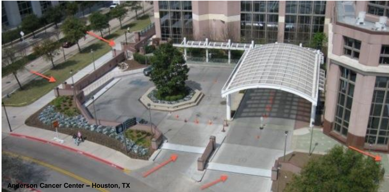
Passive flood barriers combined with garden walls
