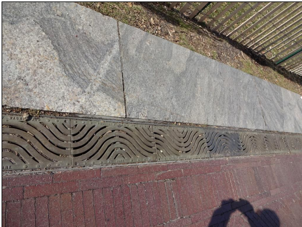
Detailed view of the drainage grates with wave pattern around the central lawn. Grates are inscribed with park name, "Robert F. Wagner Jr. Park."
