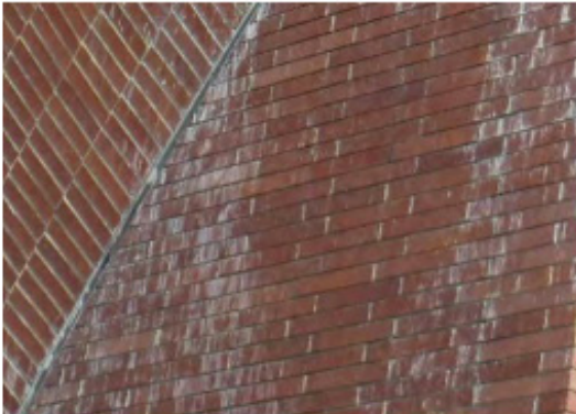
BRICK VENEER DELAMINATION, WIDESPREAD CHRONIC EFFLORESCENCE AND CRACKING
