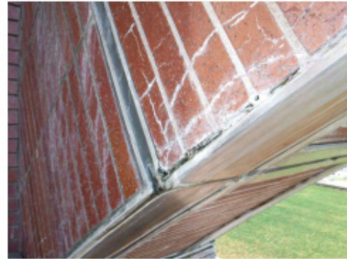
EXTERIOR NOT RESILIENT IN MARINE ENVIRONMENT AND DIFFICULT/EXPENSIVE TO REMEDiate
