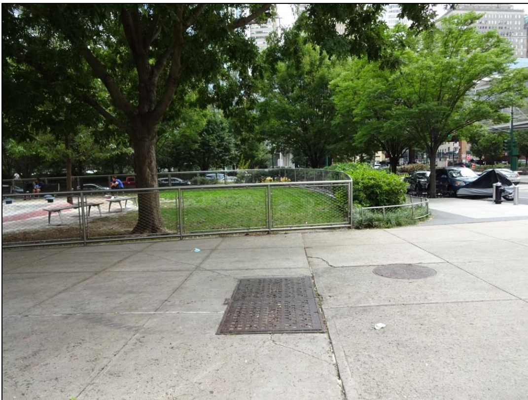
Looking east toward existing sanitary emergency overflow chamber; as part of the NSI improvements, the manhole cover would be replaced with a pressure-proofed opening.
