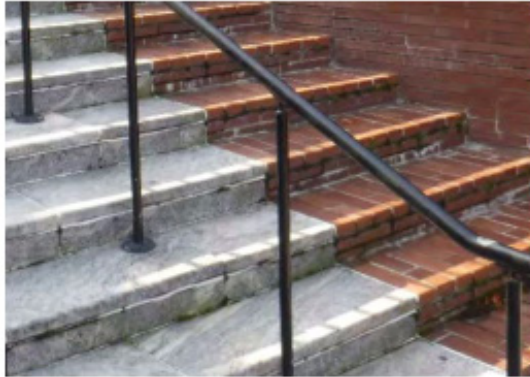
EXTERIOR MASONRY STAIRS AND PAVING IN DISREPAIR AND EXPENSIVE TO MAINTAIN
